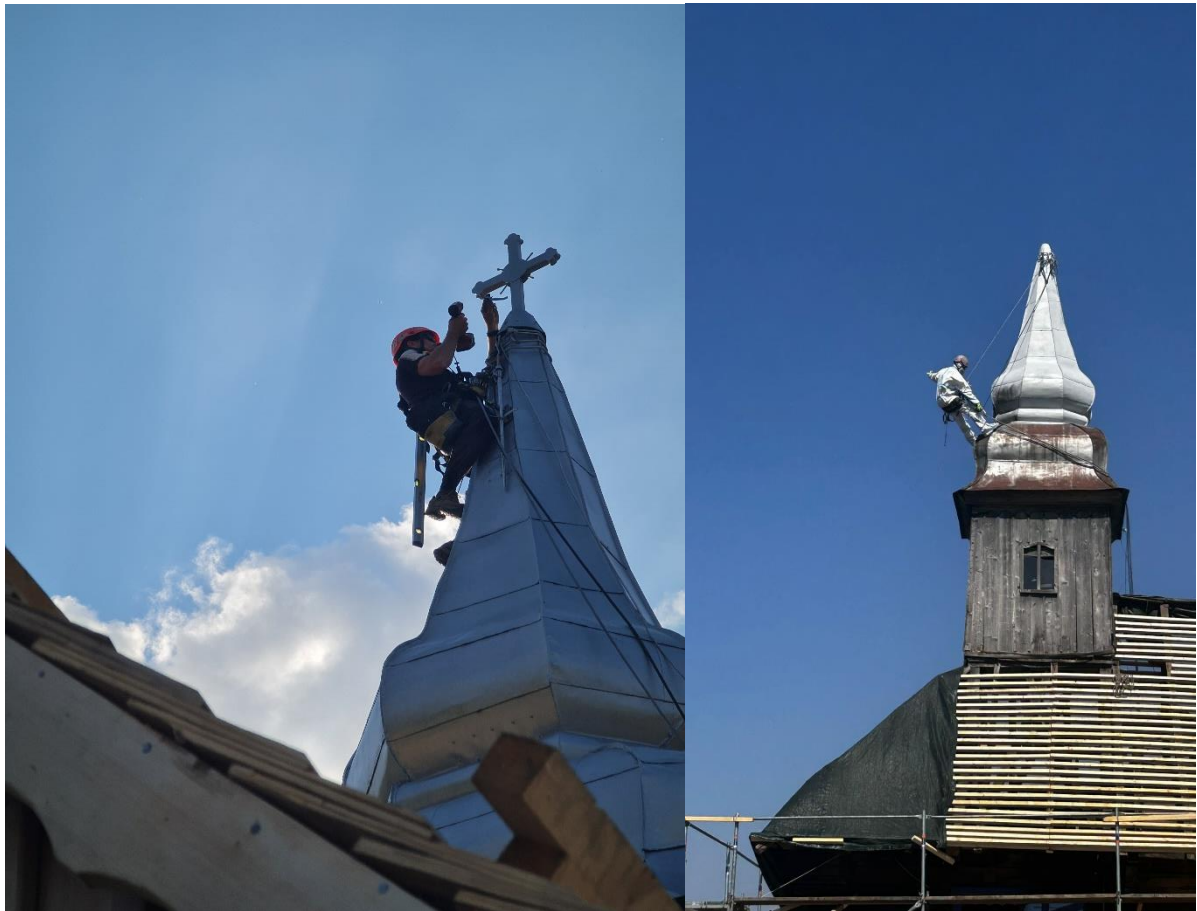
Figure 4. The industrial climber in action on the church tower.
