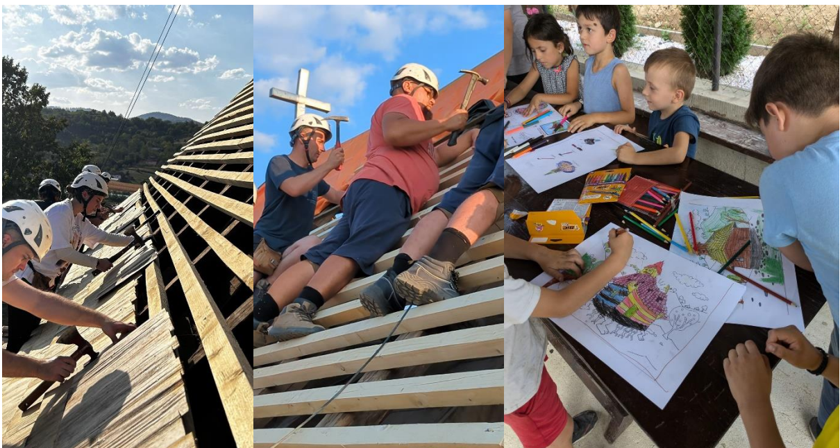
Figure 5. Left: volunteers nailing shingles on the roof. Center: the mayor working alongside the team. Right: educational activity with the village children.
