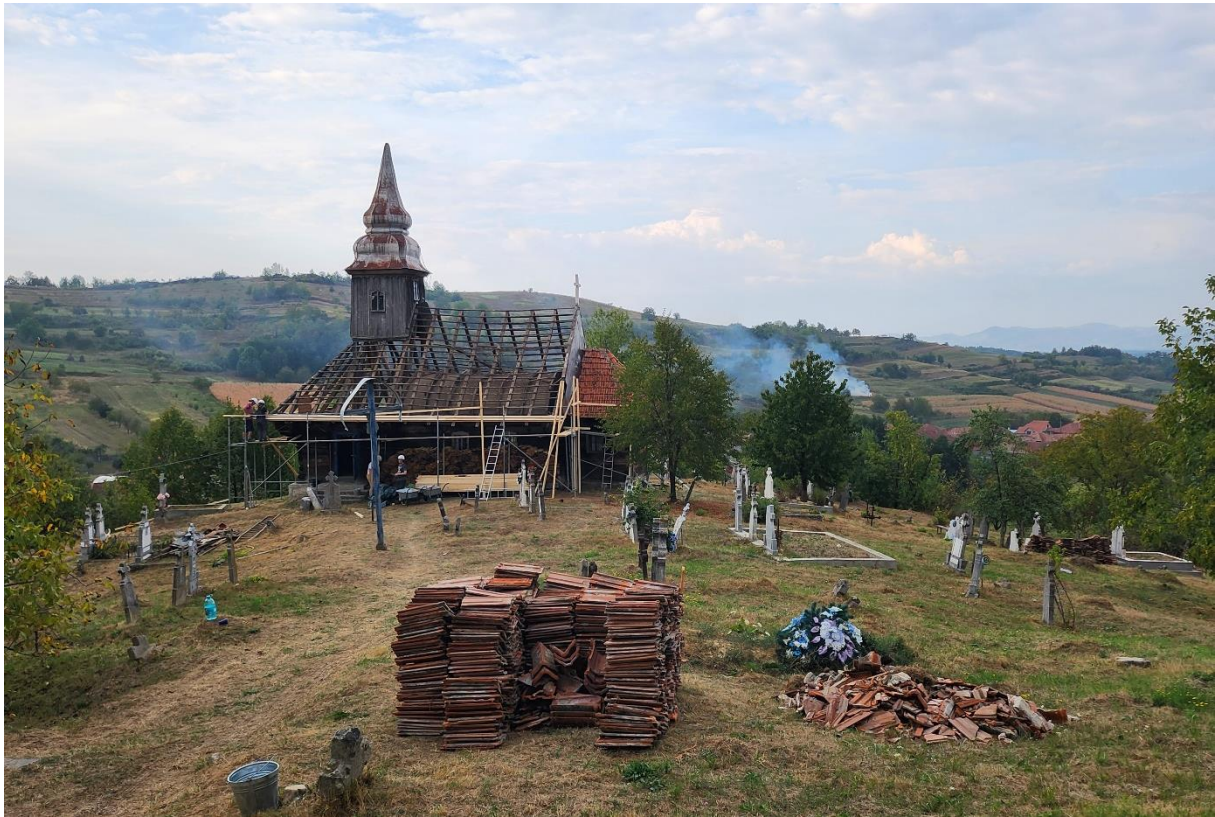
Figure 3. Transition moment: removal of the tiles and preparation for shingle installation.
