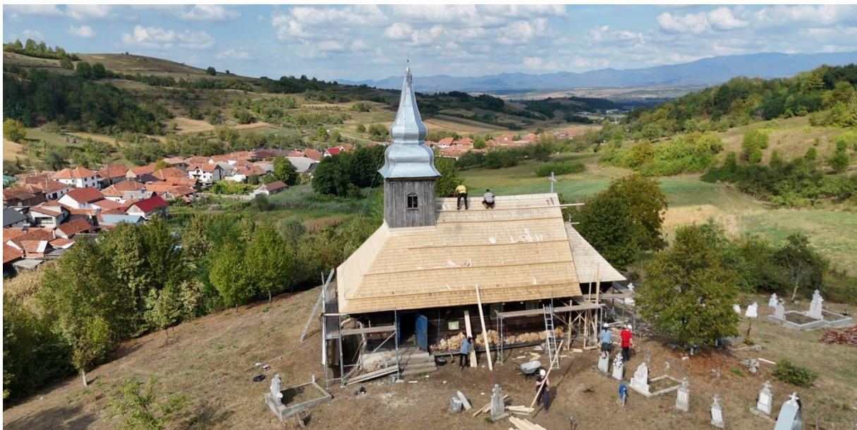
Figure 2. Aerial view of the church in Hinchiriș during the final finishing works.
