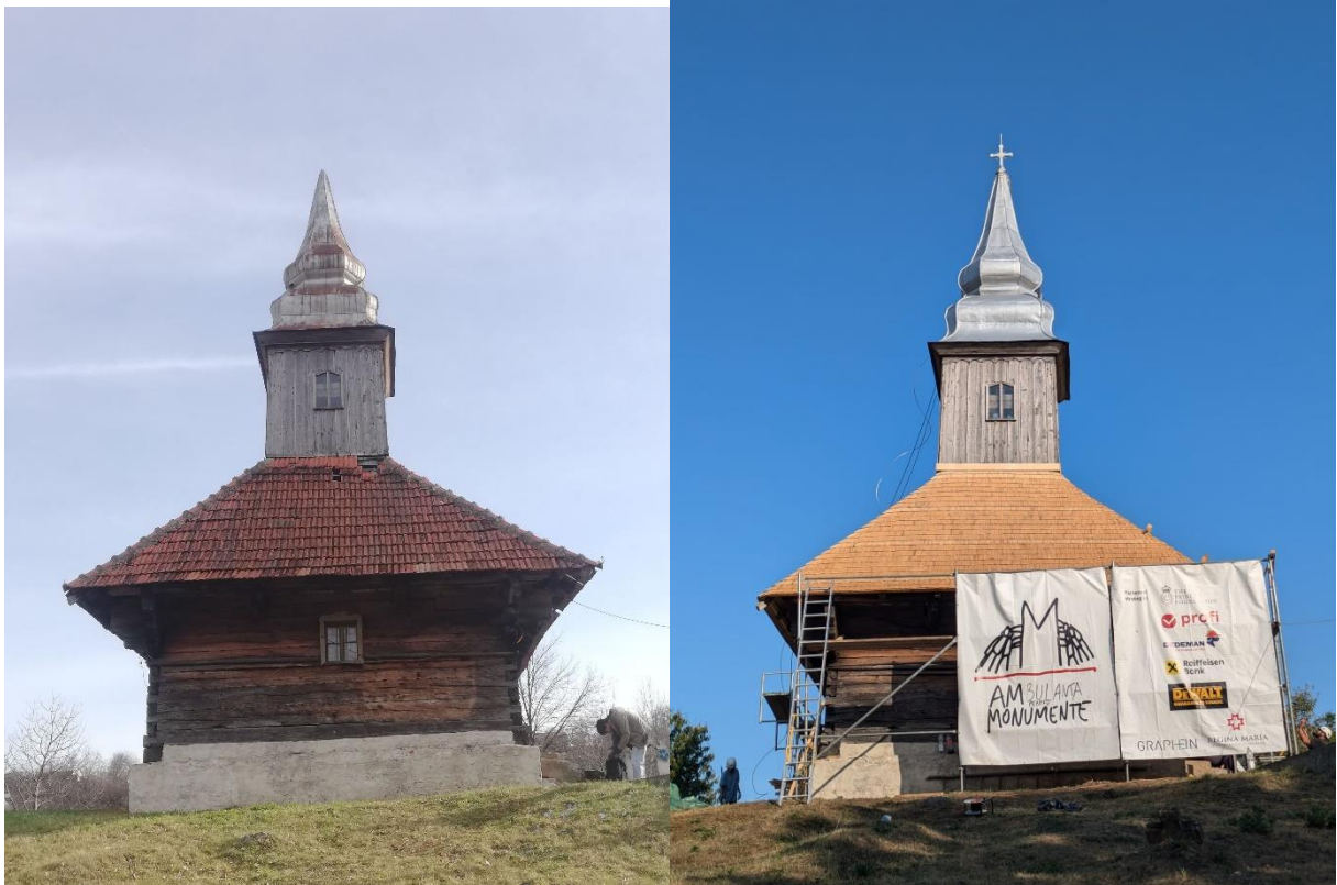
Figure 8. The transformation of the church: before and after the intervention.
