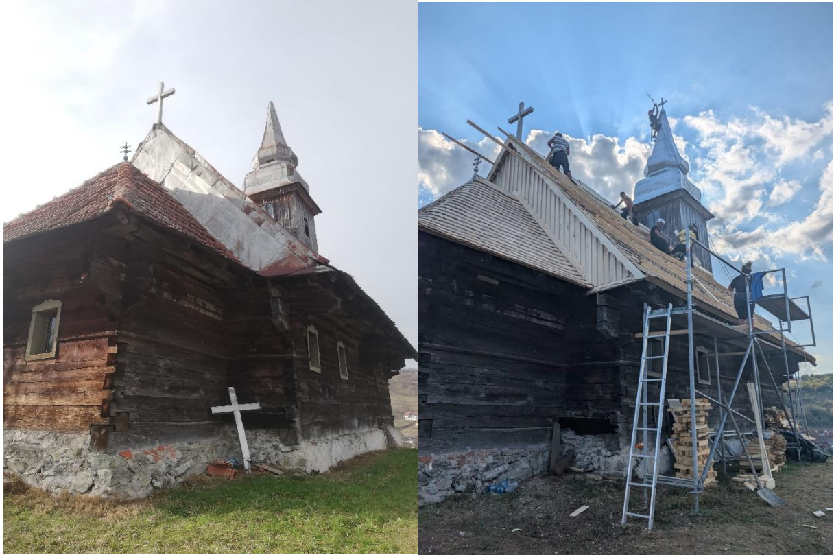
Figure 6. The transformation of the church: from the damaged roof covering to the installation of new shingles.
